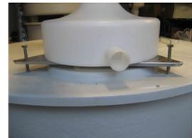
The outgoing outlet is connected to the composting chambers drainage (see the illustration on the Aquatron wagon system on the right).
